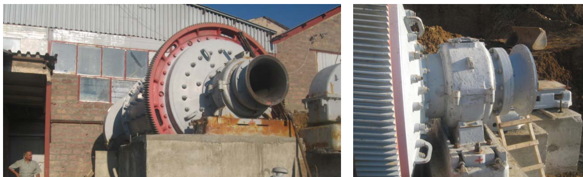
Figure 48 Installation of new mills to permit expansion of mill production Mills, outside existing mill building, on mountings ready for commissioning during October 2011 (Photos courtesy of A. Boghossian).
