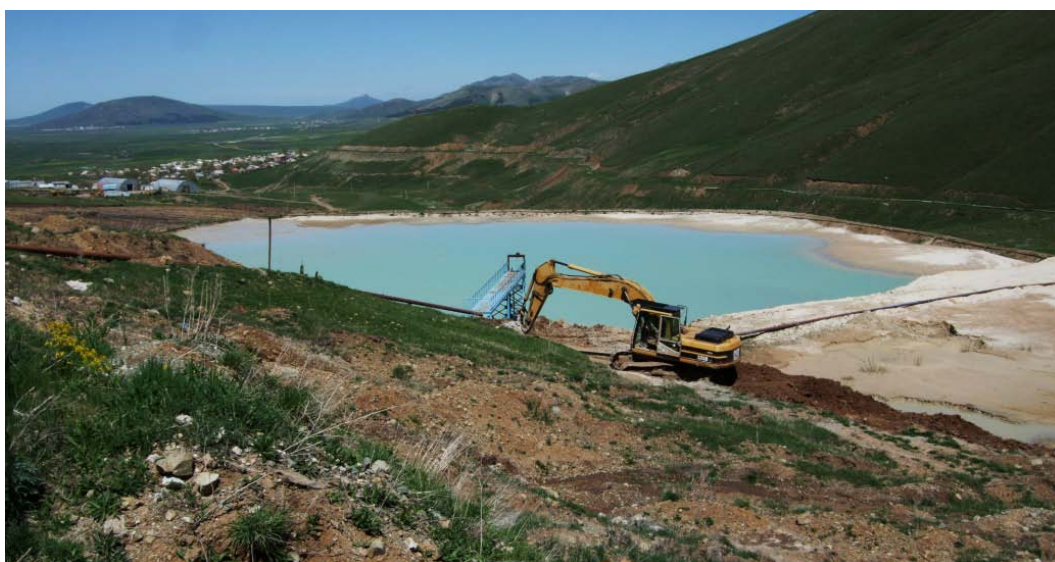
Figure 49 Tailings ponds, with discharge point Mine camp accommodation and laboratory/core shed buildings in middle distance, with pipeline route for village irrigation water supply on hillside to right.
