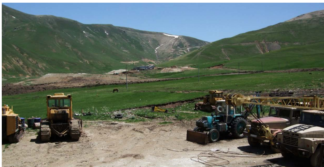
Figure 12 Toukhmanuk mine area Looking east, mining equipment in foreground, tailings dam impoundment berms and mill in the middle distance, trenches on slope of Toukhmanuk mountain to right.
