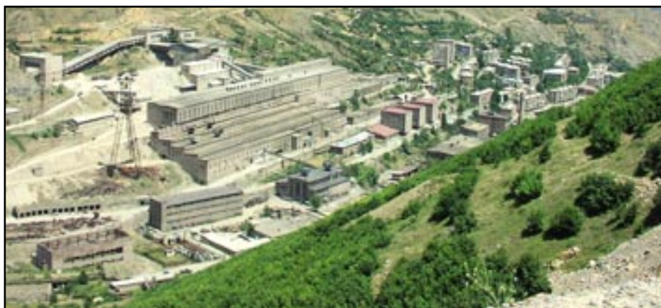
The processing plant at Kajaran, where the orebody contains 60% of Armenia's copper
